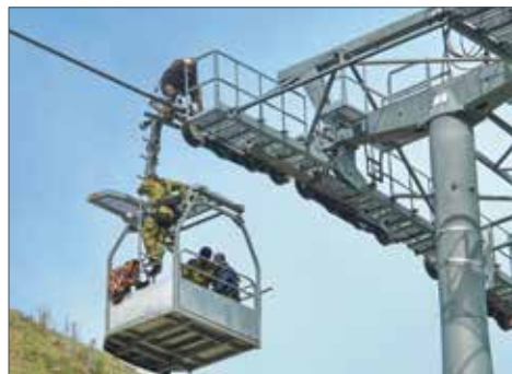
Cable car construction
